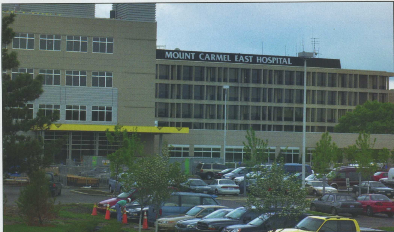
Growth in an area's medical services sometimes means growth in the hospitals themselves. Mount Carmel East is constructing a new heart hospital that will be open in 2003.
